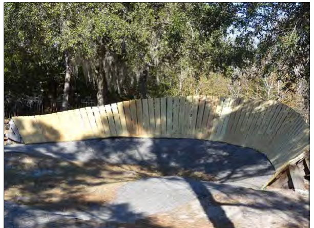
Bike Park Wooden Ramp
