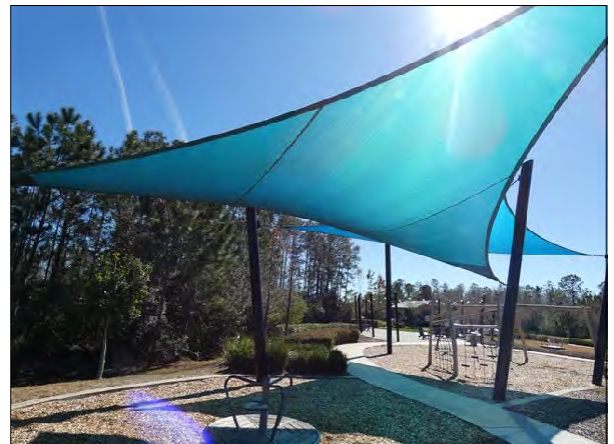
Shade Structure - Tour Trace Park
