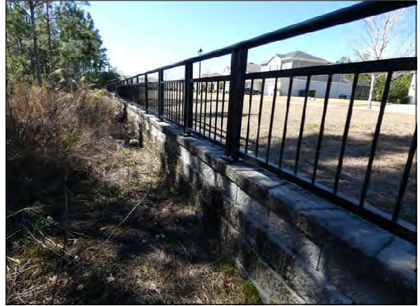
Retaining Wall and Fence
