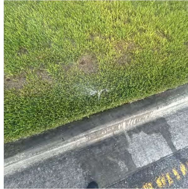
Zone #9 (Blocked Head) - 03-24-26 7:39 am CDT
