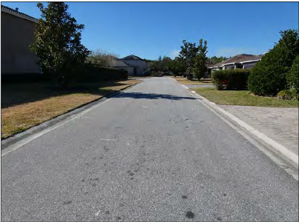
Typical Asphalt Alley
