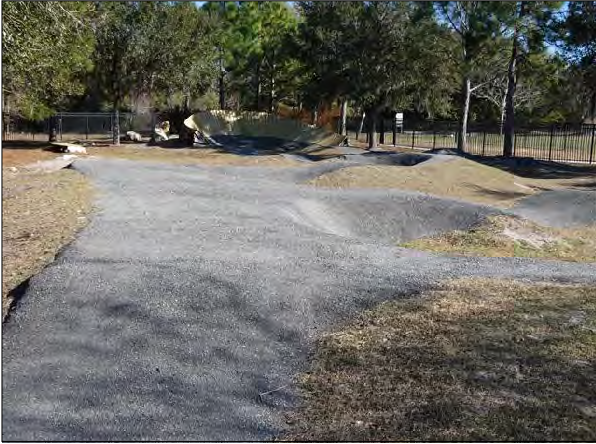
Bike Park Asphalt Surface
