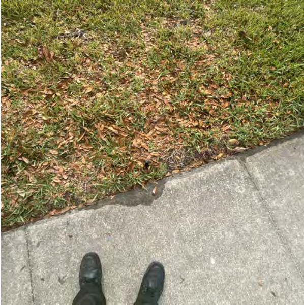
Zone #38 (Clogged Nozzle) - 03-24-26 9:43 am CDT
